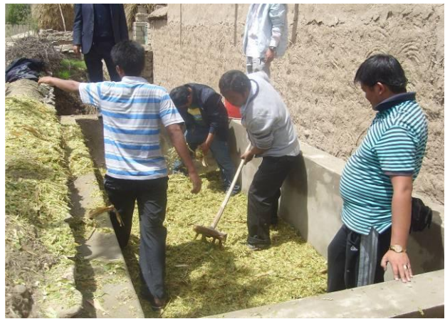
villagers are building silo
